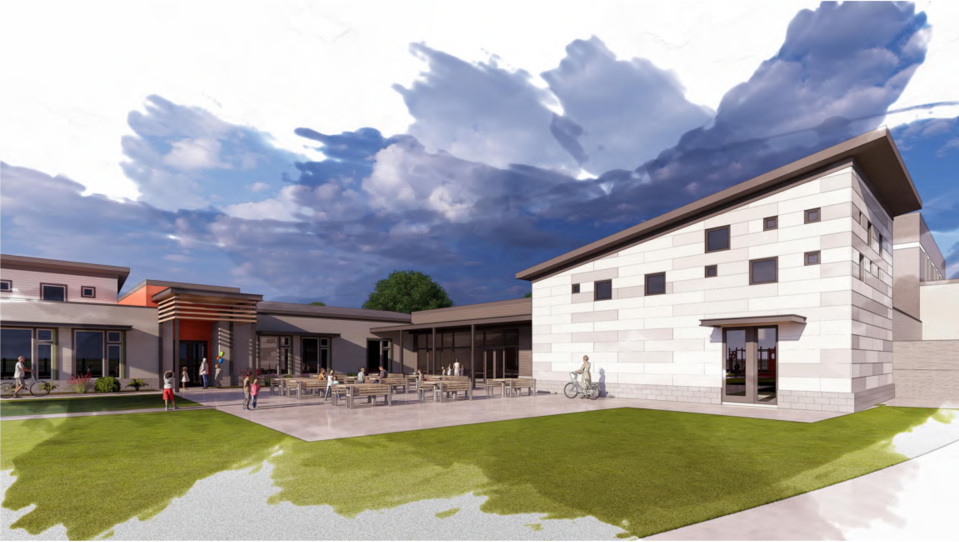
MUSIC AND COMMONS AREA, LOOKING NORTHEAST
